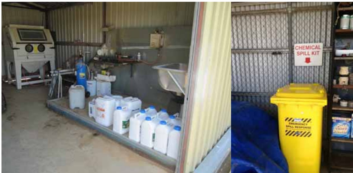
Figure 6: Appropriate bunding and a spill kit in chemical storage areas (Photos: Nina Sheer, EPA)
