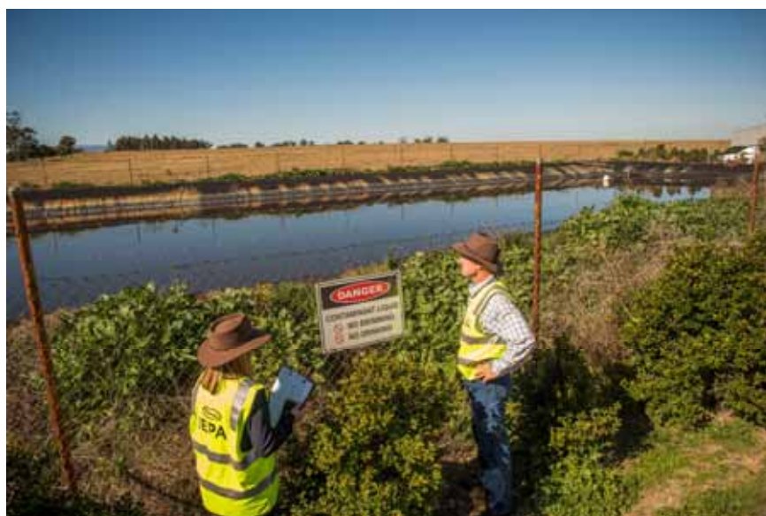
Figure 4: Lined evaporation pond with signage and fencing (Photo: John Spencer, EPA)
