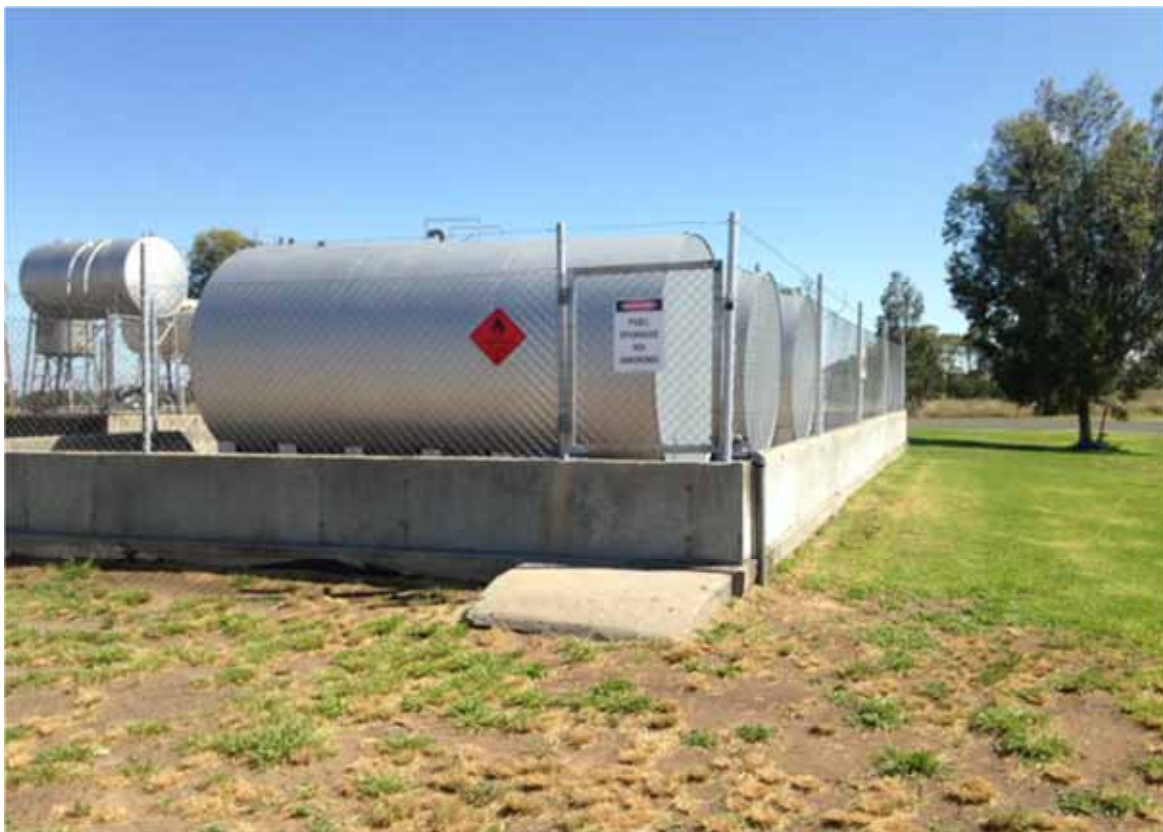
Figure 3: Example of appropriate bunding, fencing and signage around above-ground fuel tanks (Photo: Nina Sheer, EPA)
