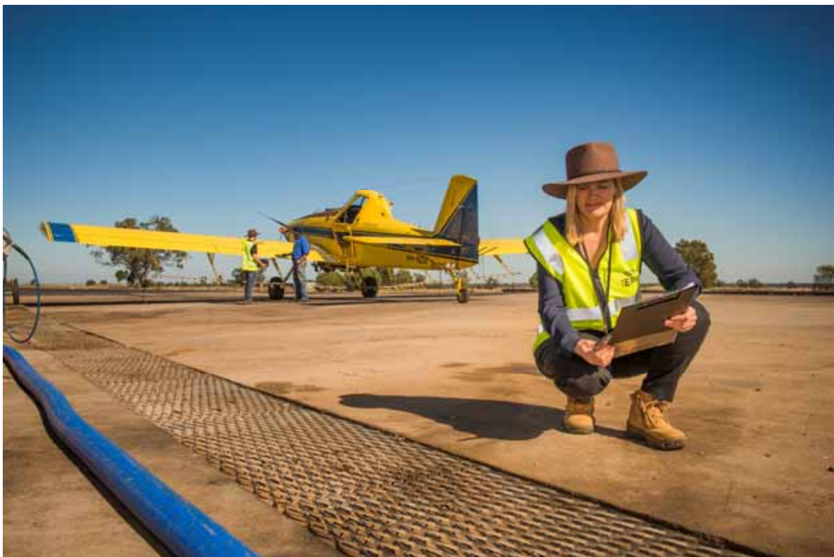
Figure 7: Open drain covered with mesh to prevent solids entering the culvert (Photo: John Spencer, EPA)
